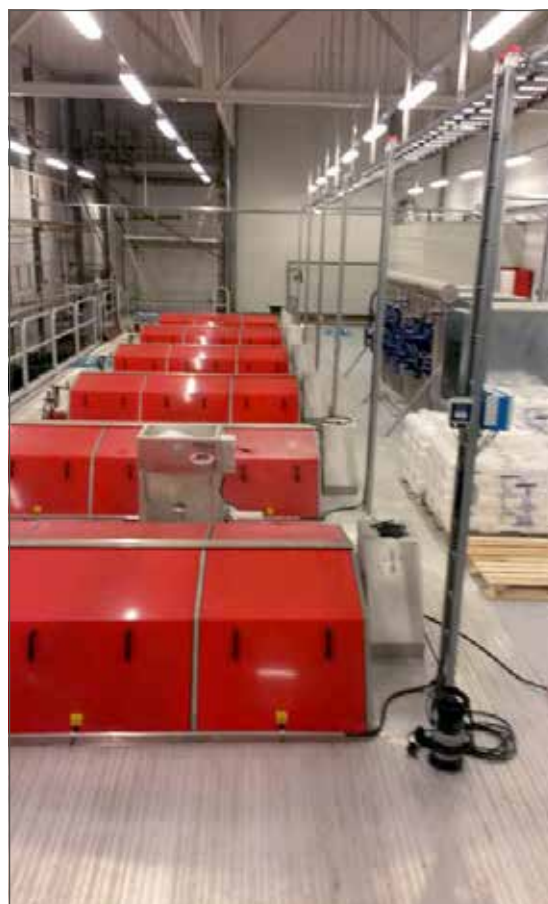
Figure 5.11. Particle removal equipment at an Atlantic salmon smolt production site. Photo: Bendik Fyhn Terjesen
