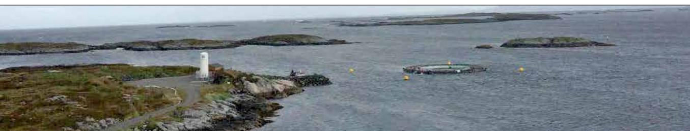
Fig. 5.19 Flexibag with the surrounding 60m sea cage at Gullklakken, Smøla (photo by Jelena Kolarevic, Nofima)
