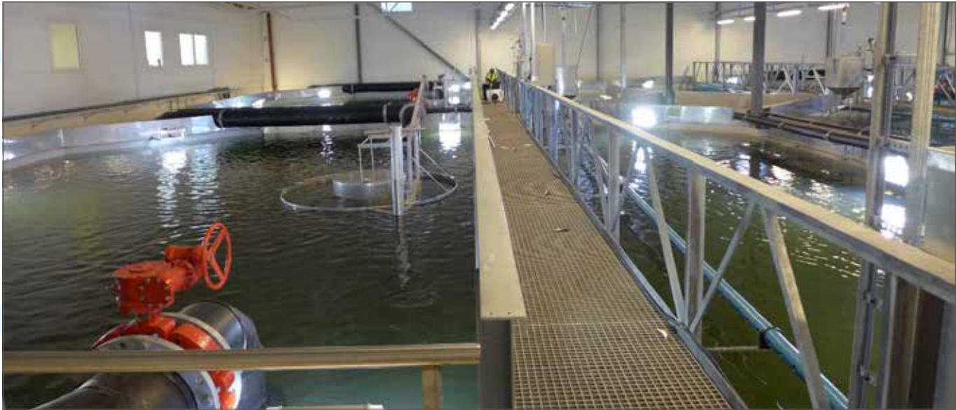
Figure 5.8. Tanks at CtrlAQUA partner site used for survey of operational parameters in the HYDRO project
