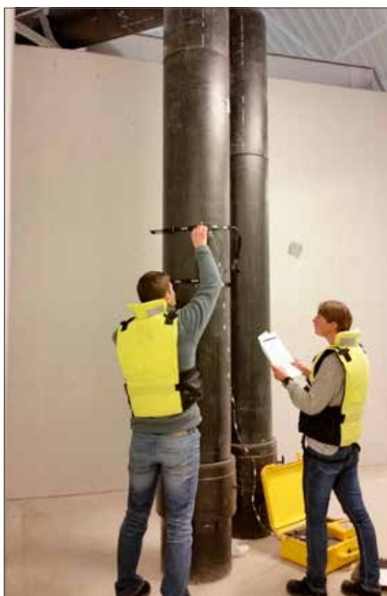
Figur 5.1. CtrlAQUA technicians from Nofima measure flow rates through intake pipes to a large-scale salmon culture tank.
