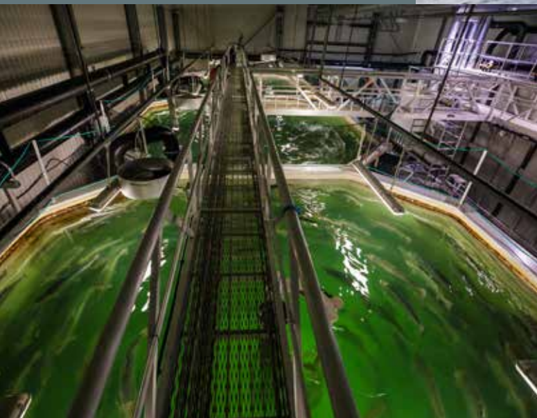
AgriMarine semi-closed containment system at Gulklakken, Smøla. Photo: Reidun Lilleholt Kraugerud © Nofima
